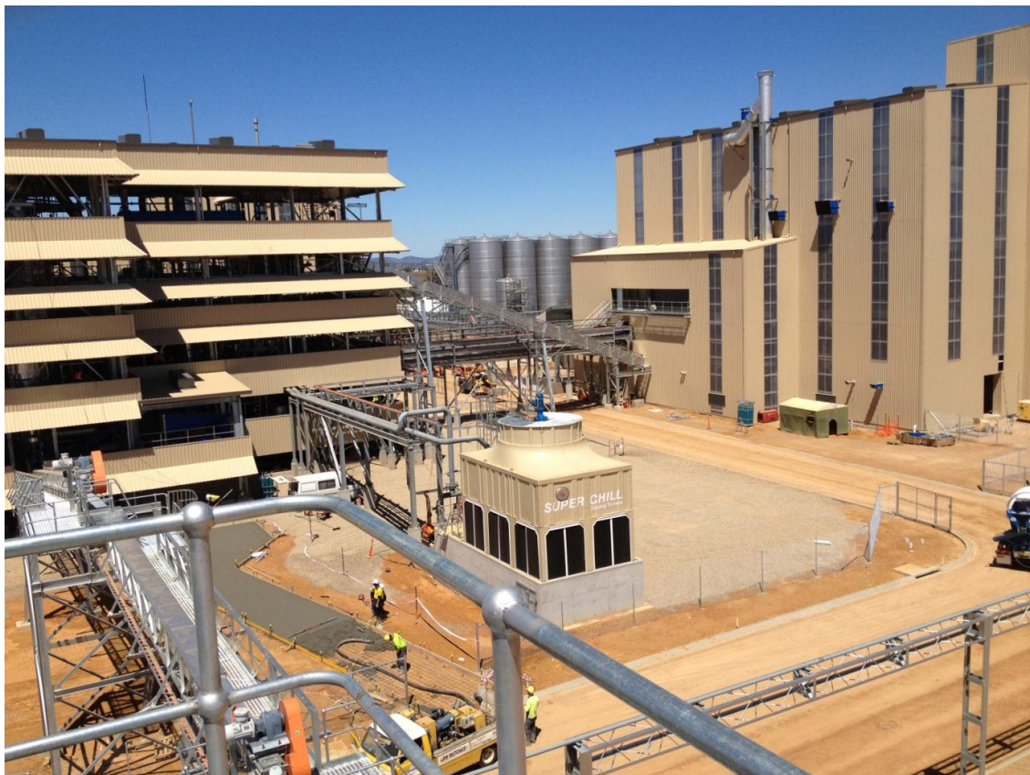
$120M Riverina Oils and Bio Energy Seed Processing Plant, Wagga Wagga NSW, during construction
